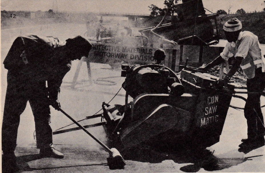
Below: a nasty skid like this is not always caused by reckless driving; the road may be at fault, not the driver. Concrete sections of M1 have recently been grooved, above and left, to improve tyre adhesion in the rain
